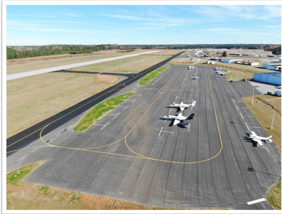
Atlanta Speedway Airport Apron Rehabilitation and Navaid Total Project Cost: $1,699,613
